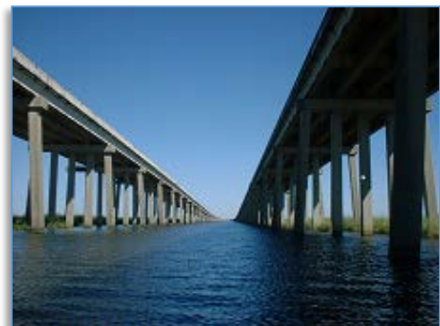
I-10 Pascagoula River Bridge
